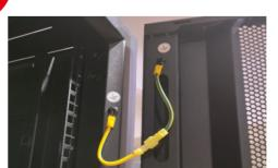
Ground wire to connect between cabinet frame and cabinet door
